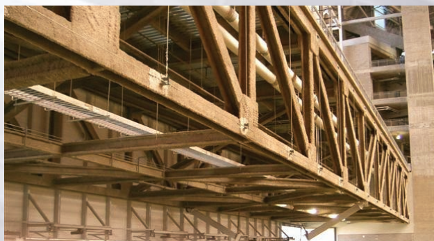
CAFCO BLAZE-SHIELD HP applied to the trusses.
