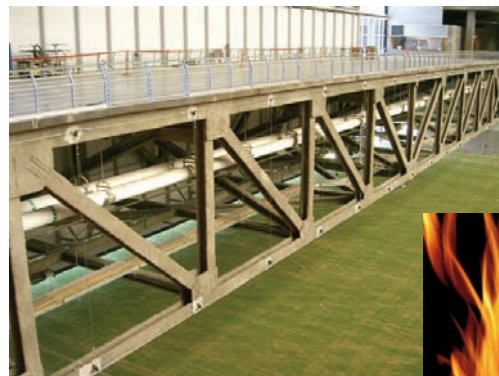
The playing field is being transferred inside the stadium past trusses fireproofed with CAFCO BLAZE-SHIELD HP.
